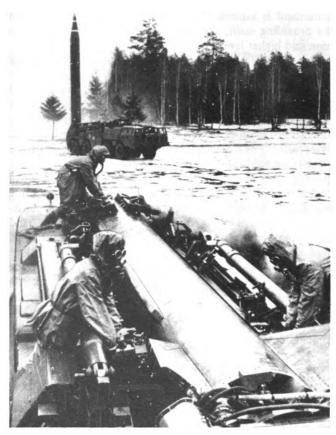
Figure 5-11. Tactical nuclear missiles. Short and medium range ballistic missiles, such as SCUD-B provide nuclear firepower at the army level. The crew, in CBR masks and protective suits, prepares to launch the missile from its mobile transporter.
